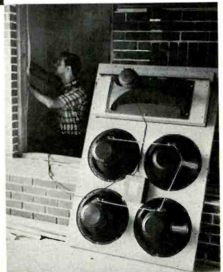
Brick-wall speaker system installation is shown at left. Various installation steps are shown below, before grille cloth covers enclosure openings.
