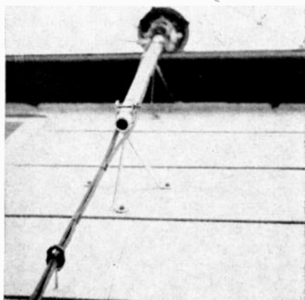
Fig. 23. Wall brackets and heavy-duty mast supporting a rotator and 10-element Yagi-Uda array. Shielded twin lead and rotator cable taped to mast and then together can be seen passing through a standoff at the bottom of the picture.
