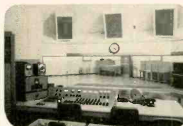
Monitoring with Altec "Duplex"® Speakers in Capitol's control room. More than 70 of these speakers are used throughout Capitol's recording studios in Hollywood.
