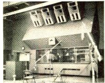
Studio A of Universal Recording Corp., Chicago, uses four Altec A-7's in monitoring 4-channel PLAYBACK .
