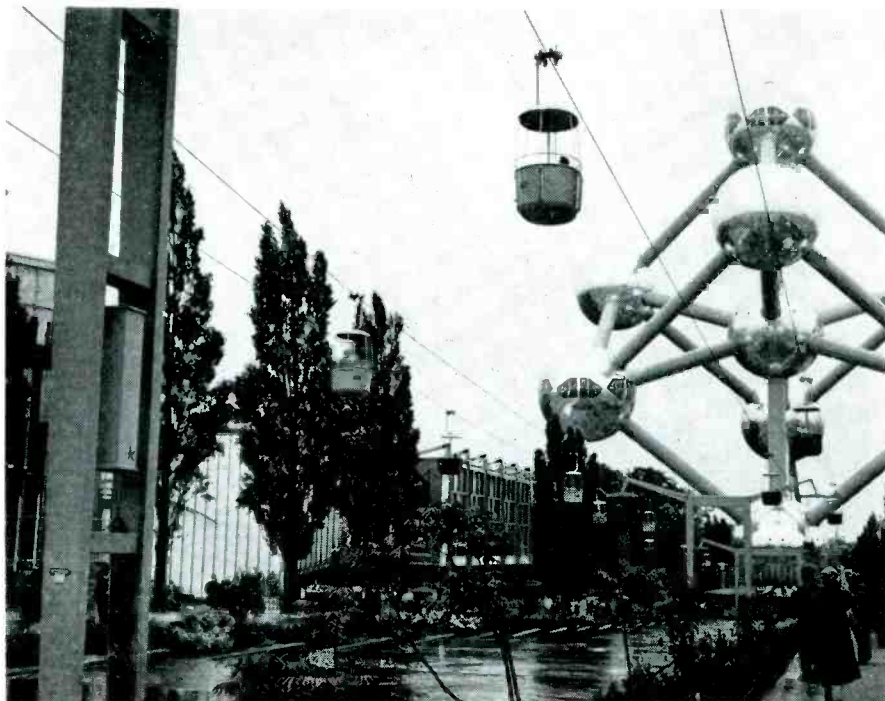
General view, showing the Atomium and the cable carriers.
