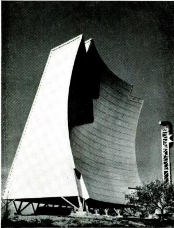
Giant over-the-horizon antenna designed by Bell Telephone Laboratories for "White Alice," Air Force Alaskan defense communications network.
