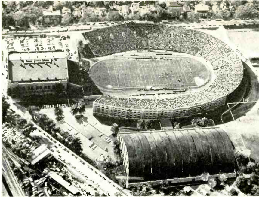
Fig. 1. This aerial view shows the stadium. The Field House is at left and the Practice Building in the foreground.
