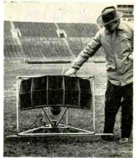
Fig. 5. Twelve of these horn-loaded speakers are around the Stadium. Mounted almost at ground level and directed slightly upward, they project sound toward the listeners who are located on the rising tiers and thence into space rather than into the town.
