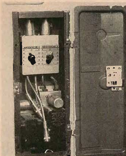
Fig. 4. Wallbox housing for small preamplifier located near the stage to feed a long line to projection room and main amplifier.
