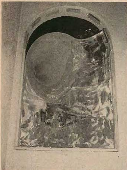
Fig. 2. Placement of trumpet horn in organ-loft opening, and fairing with plastic material to prevent reflections from inside of aperture.
