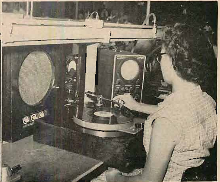
(Left) Production testing of compliance, using a magnetically driven vibrating reed which is loaded by the stiffness of the cartridge. The change in amplitude of vibration is read from the meter which is calibrated directly in compliance—the reciprocal of stiffness. A high value of compliance is necessary to prevent distortion and actual damage to the record groove. (Right) Production testing of output voltage and frequency response. Voltage output at 1000 cps is indicated on the meter while playing a test record, and frequency response is checked within a 2.5 db envelope on the face of the oscilloscope over the range from 50 to 10,000 cps. The source for this test is a sweep-frequency record.
