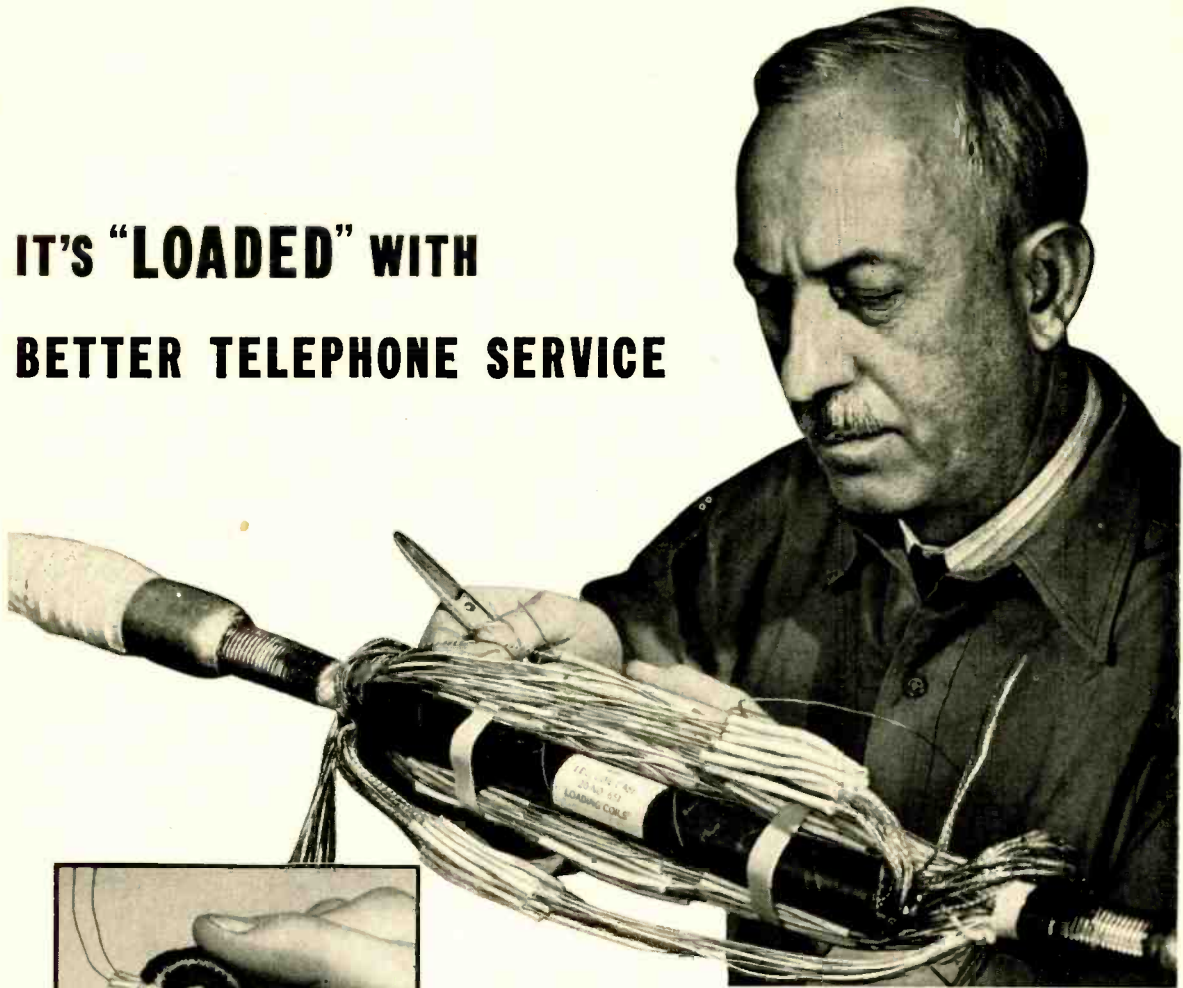
Twenty of the Bell System's newest small loading coils—like the one at the left—are housed in the long black case, mounted in a cable splice. This type of installation permits the economical extension of city cables to serve out-of-town subscribers.
