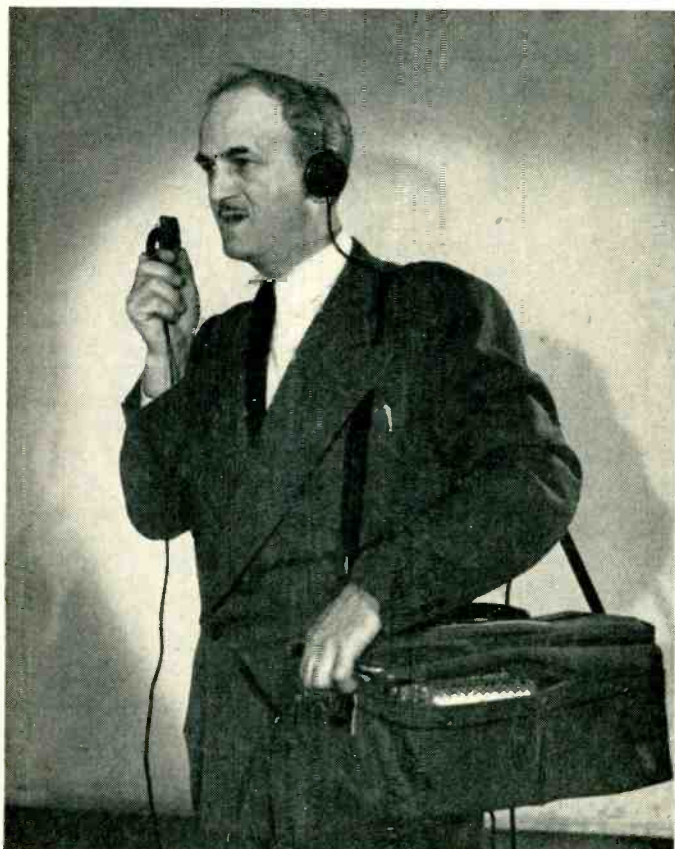
Fig. 5. The author operating a Minitape recorder. There is no level control, only a stop-start switch. The headphones monitor the incoming audio only, not the recorded tape.
