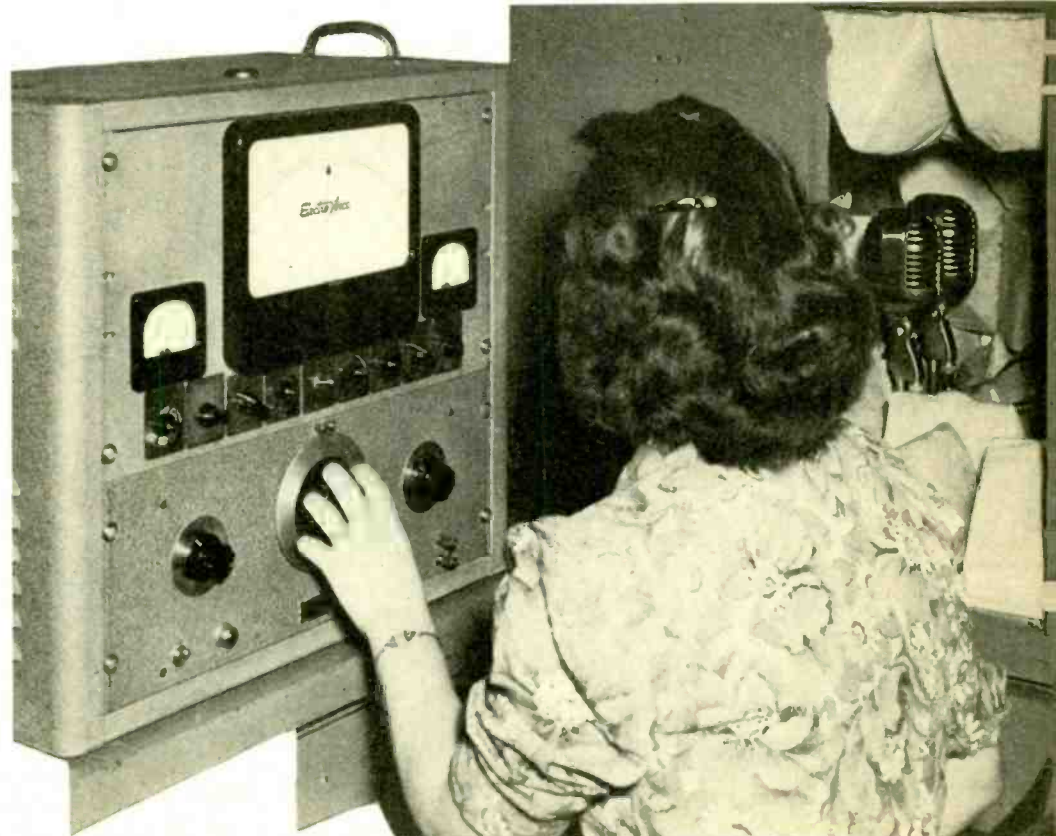
Testing microphones with the comparative decibel meter (ElectroVoice Corp.)
