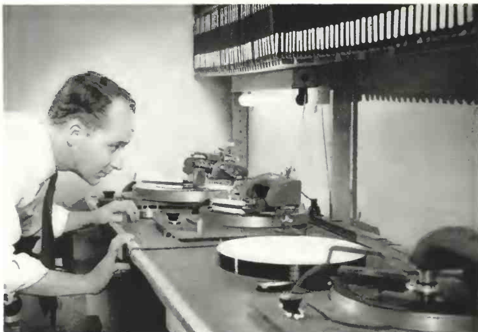
Dave Ficker keeps an eagle eye on the bank of four cutters, making acetate duplicates of a tape recording. Magnecord tape recorder is shown on the cover illustration.
