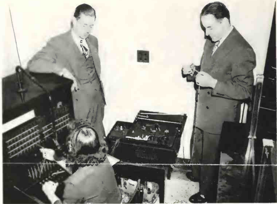
Edith Hingley, KDKA-Pittsburgh switchboard operator listens while T. C. Kenney, Chief Engineer, and J. E. Baudino, General Manager, explain the technical phases of the station's telephone answering gimmick. A magnetic tape recorder specially rigged to the outlet's switchboard played back recorded "hellos" of network stars to incoming callers—KDKA's way of hyping listener interest in web shows.
