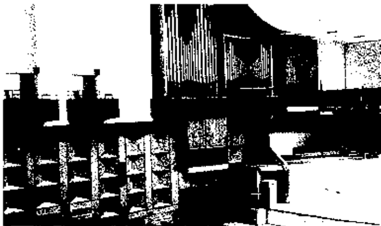
Fig. 104 Fairfield Hall. Showing the irregular alcove panelling on the side walls, the protruding columns and boxes for diffusion, and the canopy above the stage for early reflected sounds.
