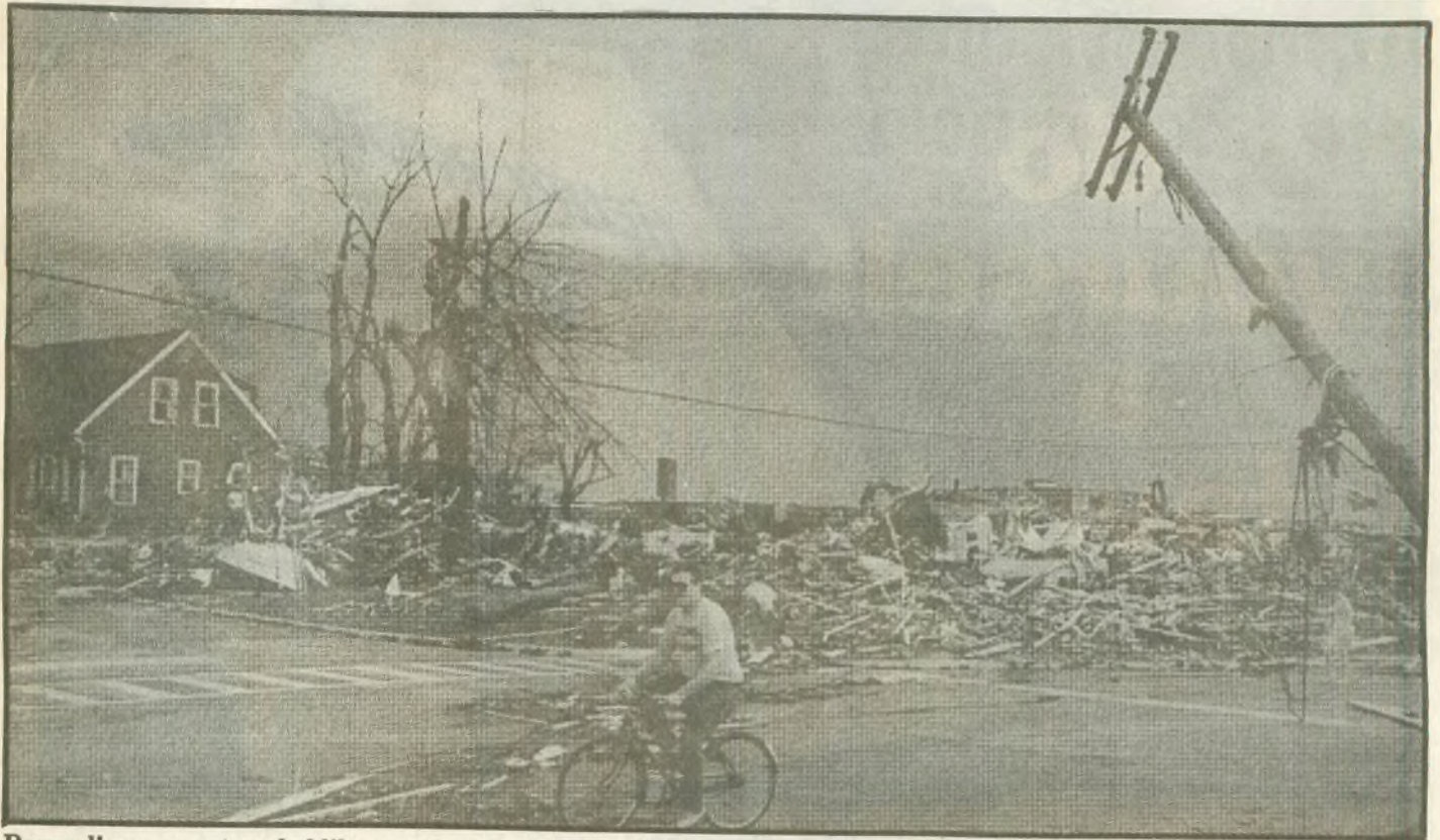
Power lines were tangled like spaghetti amid the rubble in Plainfield. (photo courtesy of the Herald-News, Joliet, IL.)
