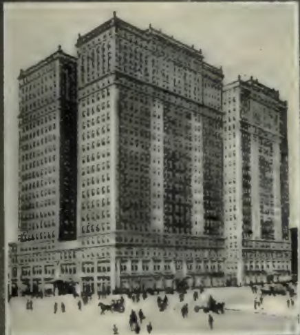
HUDSON TERMINAL BUILDING NEW YORK CITY
