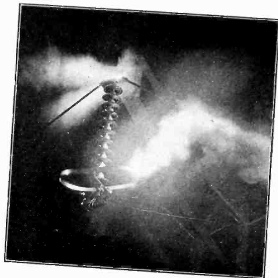
FIG. 5—FUSED GRADING SHIELD IN OPERATION DURING ONE OF FIELD TESTS
