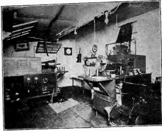
FIG. 4—INTERIOR VIEW OF WALLENPAUPACK LABORATORY
