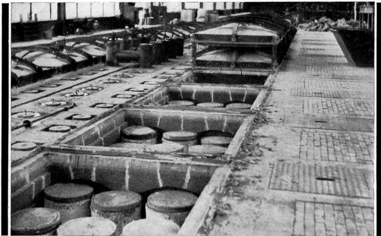
View of part of a ring furnace
