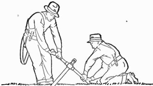
Note uncomfortable position of men screwing down old style screw anchor. Speed is retarded. Note how wrench handle catches on ground while anchor rod is still two feet above ground.
