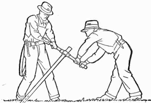
Installing new Matthews Scrulix Anchor with new style Matthews Wrench. Handle can be moved up and down wrench and set at comfortable position for men to screw down anchor. Note how end of anchor rod (shown by dotted line) is only slightly above surface of ground—anchor is down at least two feet deeper than other anchor. Men work in comfortable position during entire installation. Deeper installation means at least 50% greater holding power!
