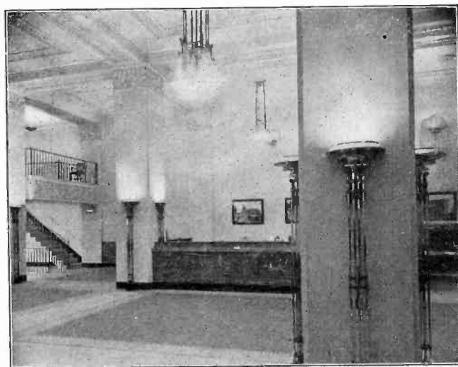
FIG. 2—A BANK INTERIOR WITH LUMINAIRES OF UNIQUE DESIGNS WHICH CONCEAL ALL LAMPS FROM VIEW
