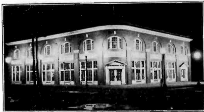
FIG. 7—FLOODLIGHTING FROM ORNAMENTAL STREET LIGHTING POSTS
