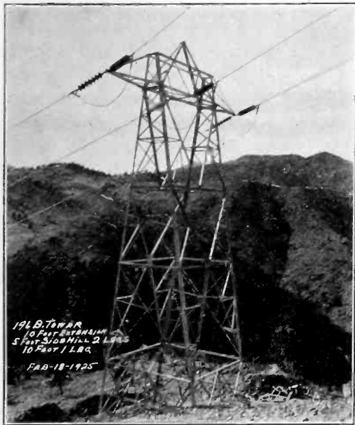
FIG. 6—TYPE OF TOWER USED ON VALMONT—BOULDER LINE
