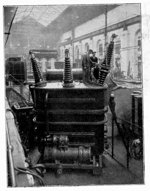
13,333 K.V.A. 110,000 VOLTS, Forced-cooled Transformers designed and constructed by FERRANTI LTD
