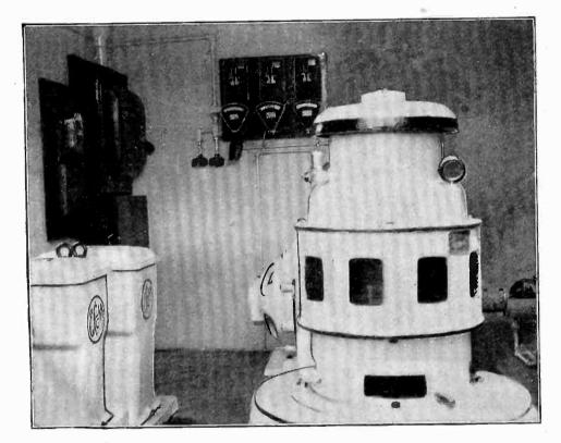
Shown above is a typica EC&M Control installation for a village water system. The Altitude Regulator starts and stops a pump through the EC&M Automatic Compensator.
