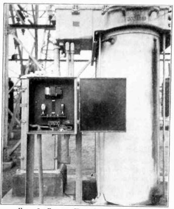
FIG. 5-DOUBLE UNIT OUTDOOR AMPLIFIER
