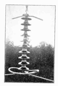
FIG. 7-RESULT OF TYPICAL FLASHOVER OF 132-Kv. IN-SULATOR STRING WITH STANARD RING AND HORN PROTECTION (Note burned ring above conductor; also horn tip slightly burned. Insulator undamaged)
