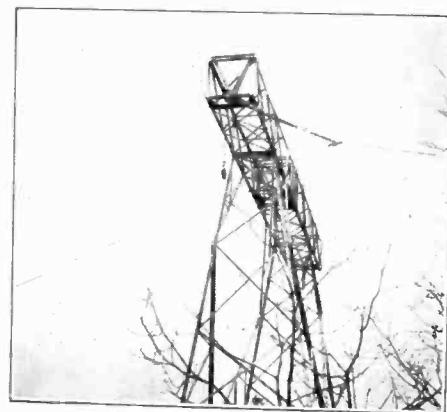
FIG. 11—TOWER NO. 1 AFTER "CUT" SHOWING DUMMY INSULATOR EMBRACING SPRING DYNAMOMETER AND IMPACT DYNAMOMETER
