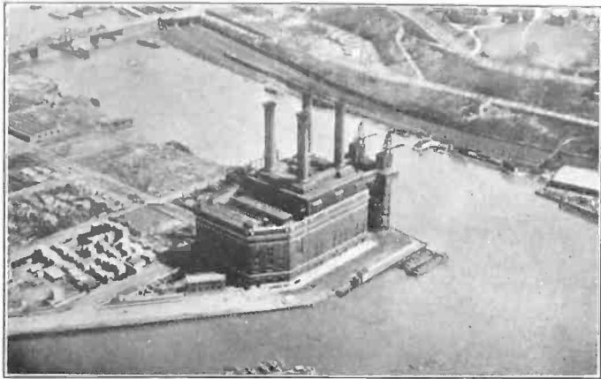
SHERMAN CREEK STATION OF THE UNITED ELECTRIC LIGHT AND POWER CO.
