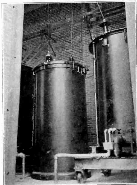
FIG. 14—VIEW OF REACTOR INSTALLED
