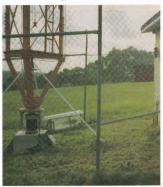
Main 135m radiator showing base insulator and grounding system.
