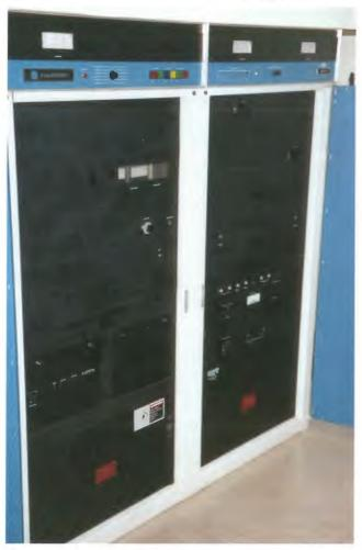
One of a pair of Harris 10 kW transmitters derated to 5 kW.
