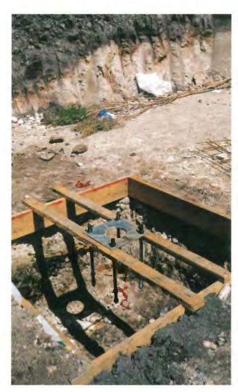
Mast thrust block formwork and steelwork in place, Strahan.
