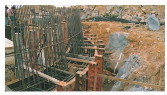
Close up view of reinforcement and ring beam formwork.
