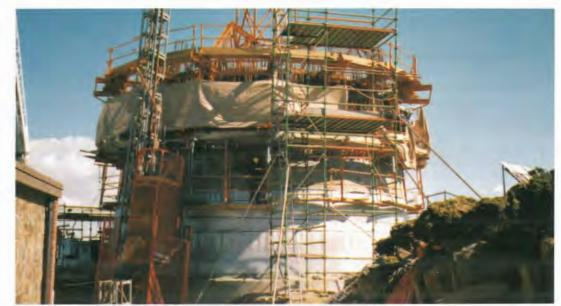
Slipform at RL 5.0m and progressing upwards.
