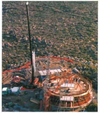
Final stage of slipform assembly and adjustment.
