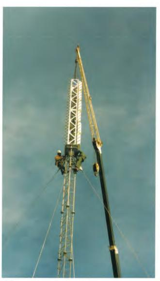
UHF antenna being placed in position on mast at Taroona.
