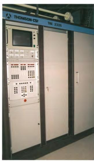
Transmitter control panel and video colour display module.
