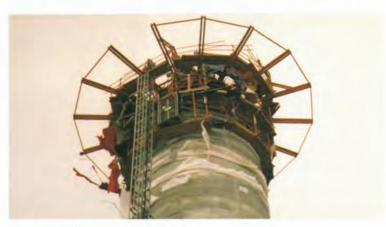
Close up view of slip form and hoist guide frame.
