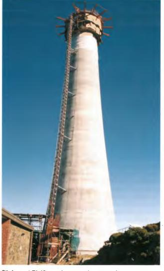
Slipform at RL49m and progressing upwards.
