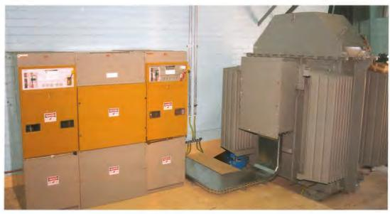
11kV switchgear and 11kV/400V step-down transformer.
