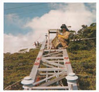
CO2 lan Tyers welding at the top of one of the power line towers.
