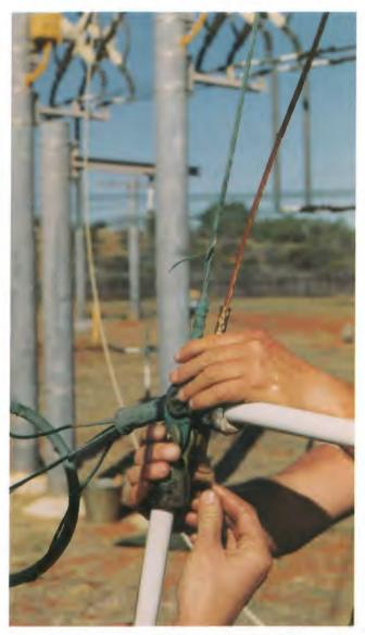
Preparing to patch-in replacement copper wire lead.
