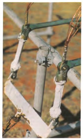
Insulators coated with high voltage silicon grease compound.
