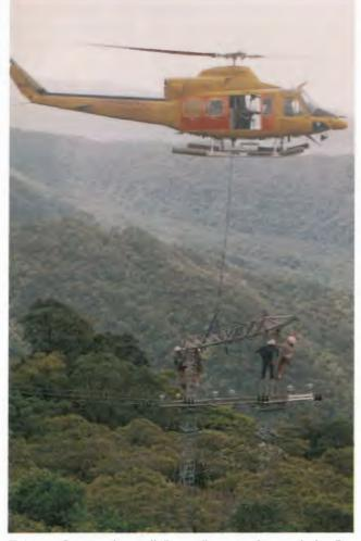
Telecom Construction staff dismantling part of transmission line tower as helicopter prepares to lift away a section.
