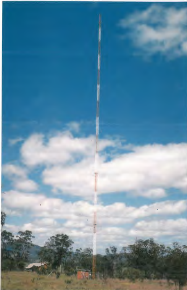
One of the two 92 m masts. Transmitter building in background.
