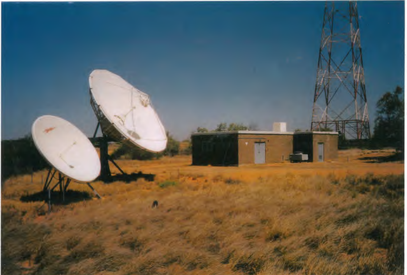
L to R. NTA dish, GWN dish, SPAN building with old Optical Telescope pedestal on roof, tower No 1 Radio Australia aerial system.
