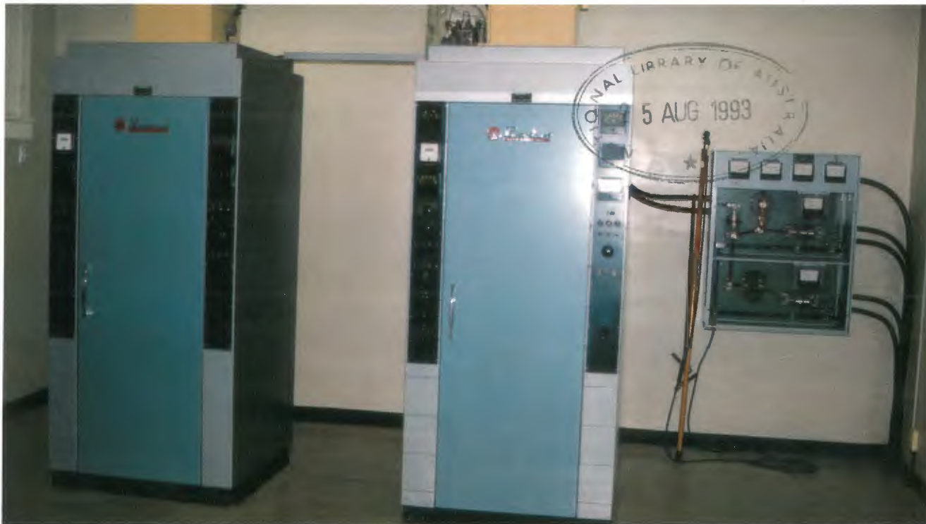
AWA BTM2-5 transmitters installed 1975
