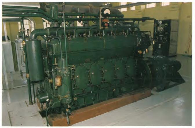
The 6 cylinder Ruston and Hornsby diesel generating set. Part of the original 2CR Cumnock 1937 installation.
