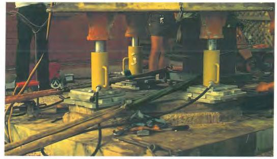
Replacement base insulator being pulled into position.
