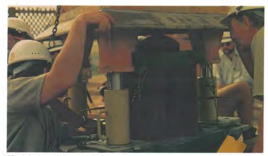
Mast being lowered on to new insulator.
