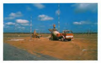
Mixing of concrete on site using modified delivery truck. Dave Arrattz on truck and Ray Hunter with front end loader.
