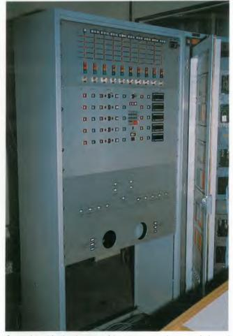
Control and indicating panel for antenna selector switch and power system during installation.
