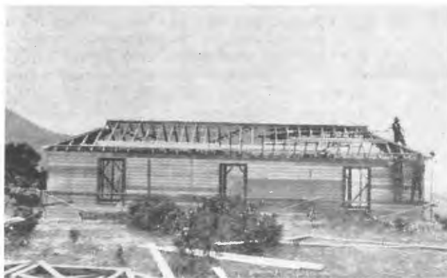
7ZL transmitter building during erection at Radio Hill, December 1926.
