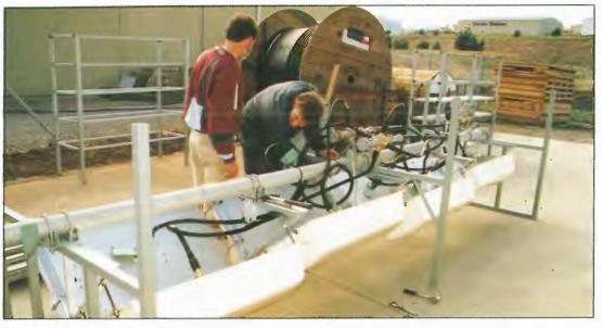
Assembly of a 2 sided UHF panel array.
