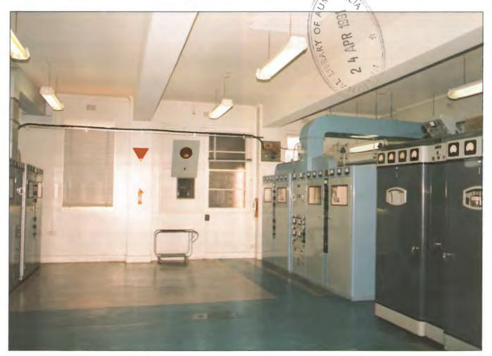
Present Canberra transmitting centre. (Far right) 2CY 10 kW. (Right) 2CY 2 kW standby also used for Radio for Print Handicapped service. (Left) 2CN 2 kW transmitter.
