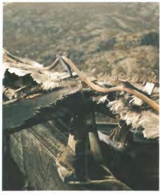
Damaged fibreglass on radome top.
