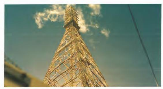
The Mt Canobolas tower showing VHF batwing antenna system.
