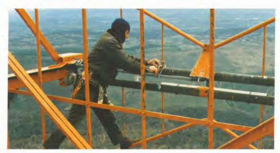
Ross Clugston CO2 dismantling deicing cables on batwing antenna.
