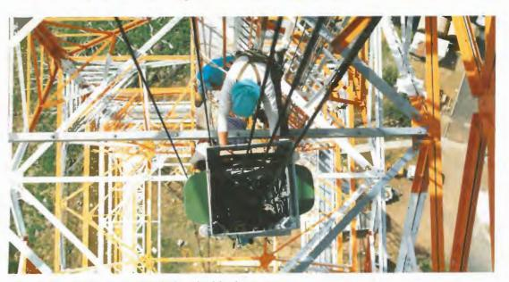
The UHF antenna being hauled up inside the tower.
