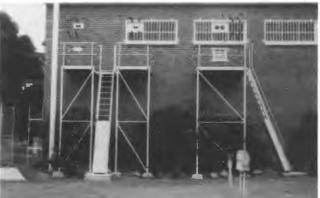
*Line termination access platforms showing barred access step covers.*
