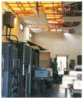
Damage to ceiling and roof of transmitter building.
