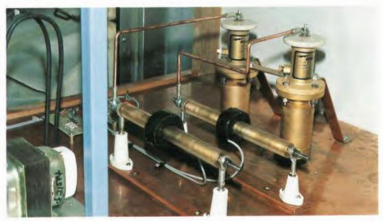
Cable terminations and line current transformers - 4CH.
