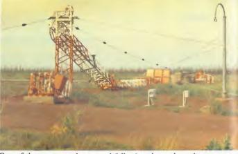
One of the masts on the ground following the cyclone damage.
