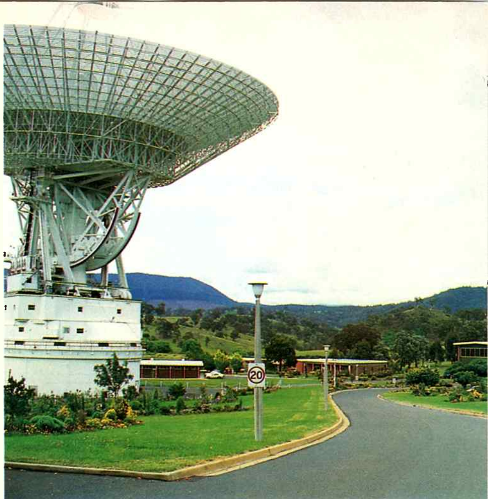
The Tidbinbilla tracking station is one of three that make up NASA's deep space network.
