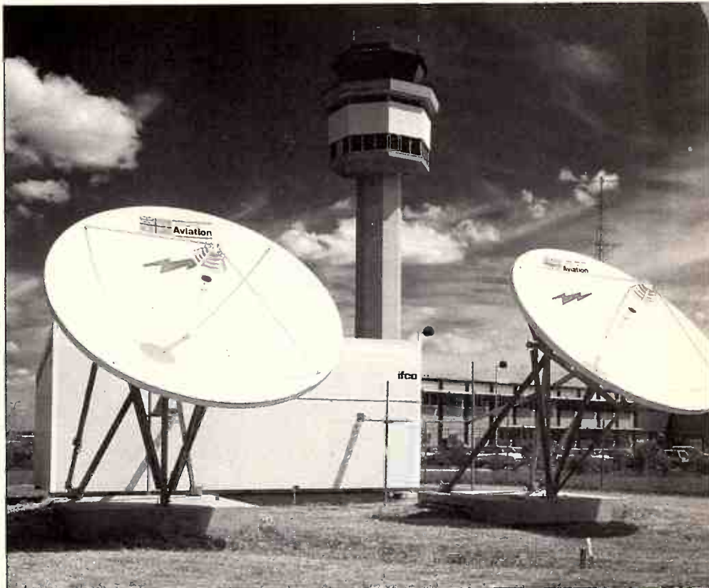
The Department of Transport was recently faced with the enormous challenge of installing 150 Aussat satellite terminals throughout Australia.
