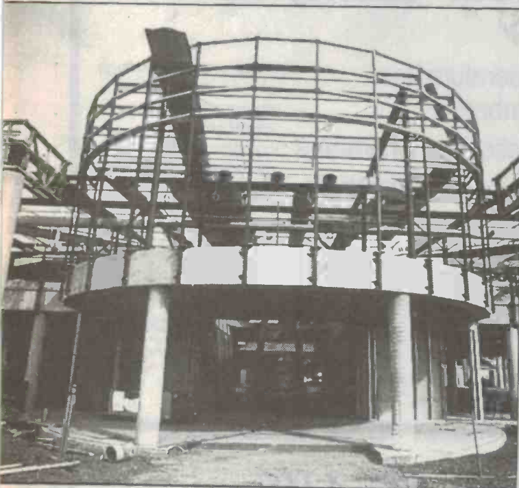
At the SA Technology Park British Aerospace headquarters are under construction.
