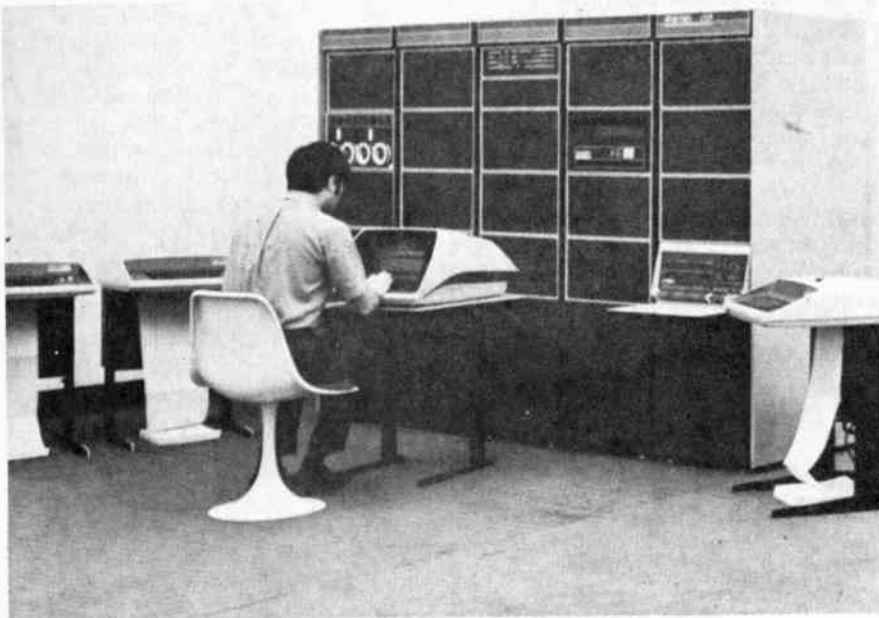
A P.D.P. 11/45 Computer System, similar to those to be used for Control and Data Acquisition in the Gladstone Power Station.
