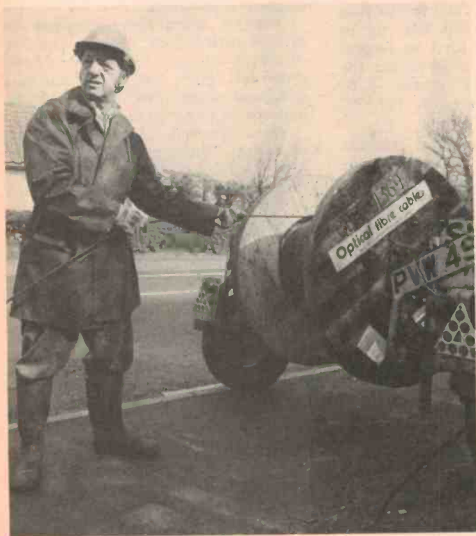
Left: Installing optical fibre in telephone cable ducts for a trial in England. (Picture courtesy of the BPO). Below: One of the regenerative receivers used in the Frankfurt region.
