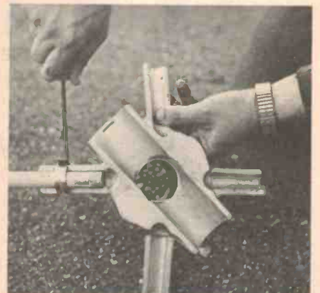
Secure each spreader with a hose clamp. Butt the end against the lug on the casting.
