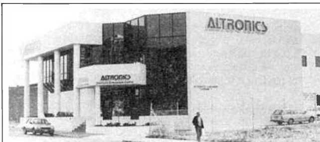
Altronic's new headquarters is located at 174 Roe, Perth, right on the edge of Perth's central business district, across the railway line from the Entertainment Centre. It houses their retail store, warehouse and administrative operations and features off-street customer parking. The building is all-white with prominent columns at the front, giving rise to its local nickname of the "Taj Mahal".
