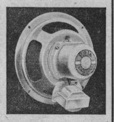
Illustrated is the Rola Model DP5B, which has been used for the new 4/38 Dual Wave Receiver, It is specially suited to the requirements of this set, and it incorporates the patented Rola dust-proof and acoustic filter assembly.
