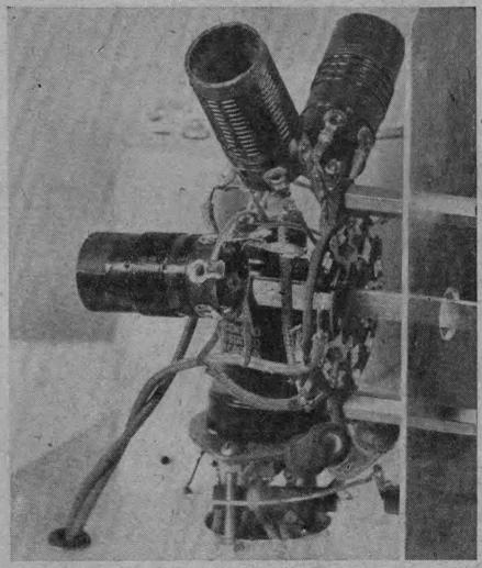
A close up of the detector grid coils of the 2JU Special Five. Note the aerial leads running through the chassis for doublet connection. Various matters of layout and mounting are illustrated hers. Note the mixer value in the background.
