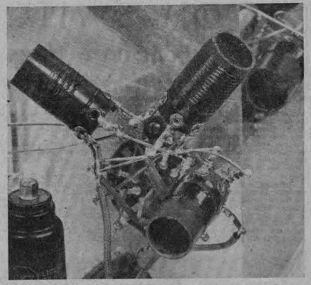
Another view of the 2JU Five detector section. The oscillator section is in the background, partly obscured by the shield. The detector valve we were using when this picture was taken happened to be a 6K7 in place of the 6L7 specified.
