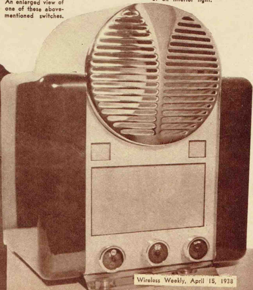
Below: A curious and interesting cabinet made all in metal. See the new switches which show the position of the various wave-bands by means of an interior light.
