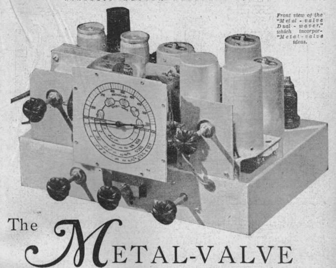
The new metal valves, together with many other modern ideas, go into this set to provide an exceptional performer for the advanced experimenter and the trade technician. A system of reflexing is used which provides two effective stages of intermediate amplification, together with a high-gain audio stage, yet there are only six valves in all.
