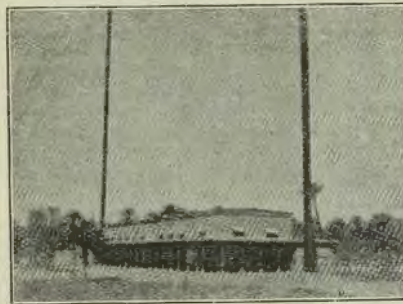
30-Kilowatt Station used by Indian Government for communication between larger cities.
