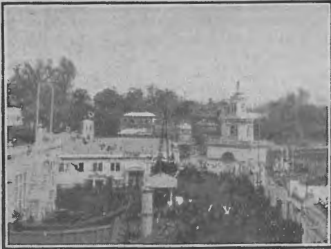
ELECTRICAL EXHIBITION. MAIN ENTRANCE.
