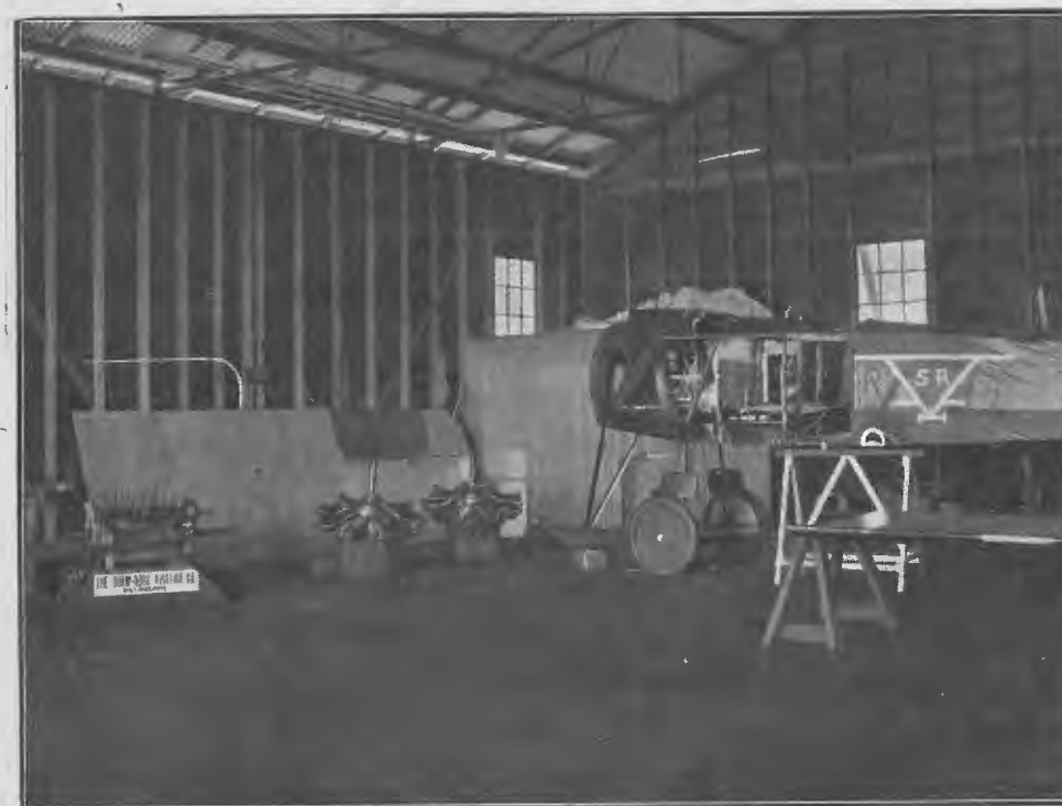
Interior View of the Workshop.
