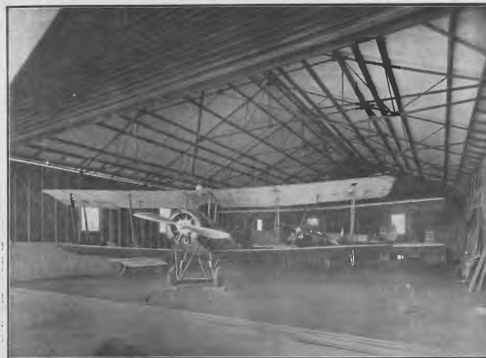
Interior View of the Hangar.
