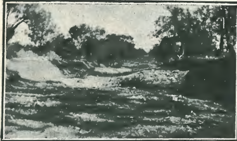
Main Road, Benalla-Wangaratta.
