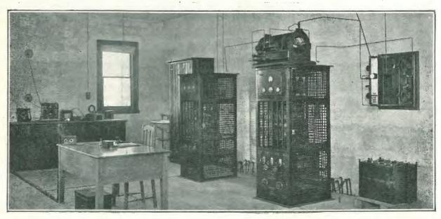
A corner of the station's operating room. On the right is the 2 Kw. Oscillator Panel, while further back is the Modulator Panel,
