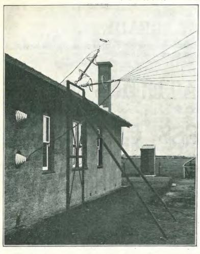
A close view of the aerial lead-in and counterpoise systems. Note the large insulators.
